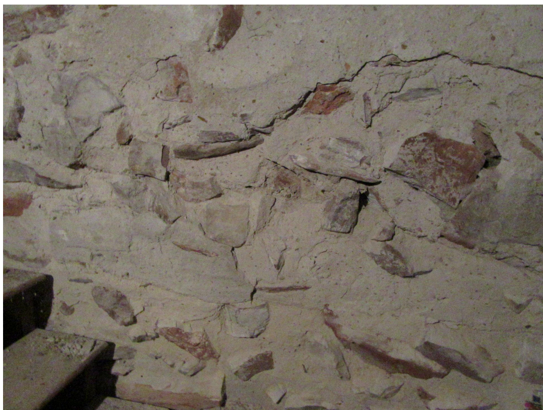
Basement foundation. Some areas were reconstructed with brick after the Fiesta Theater fire.
