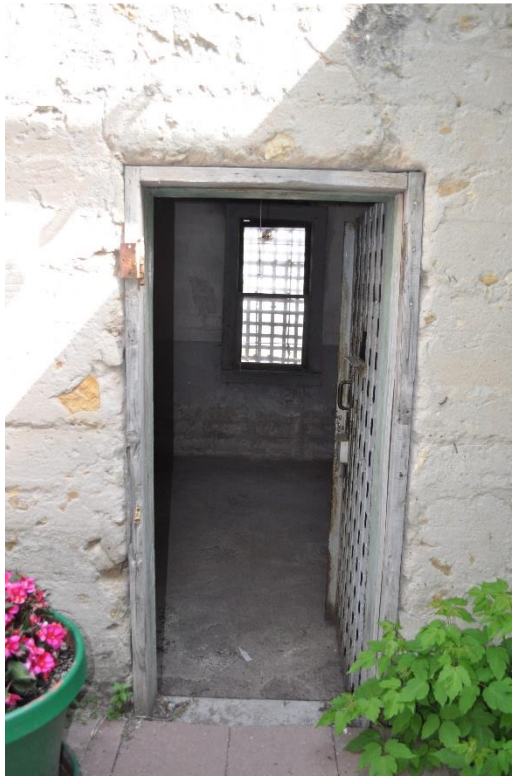
Entrance to the 1911 jail at 219 S. Gillette Avenue.
