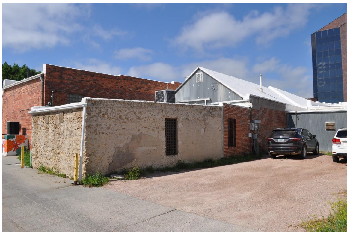
219 S. Gillette Avenue as seen from the alleyway behind the building. The change in the roof level seen above the black vehicle shows where the original roof was extended in the 1950s.
