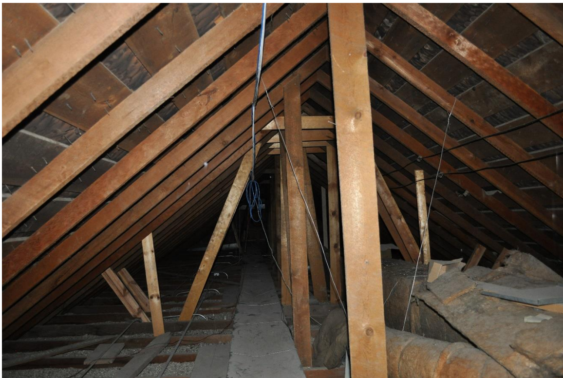
Attic space over the original 1898 section of the building at 219 S. Gillette Avenue.
