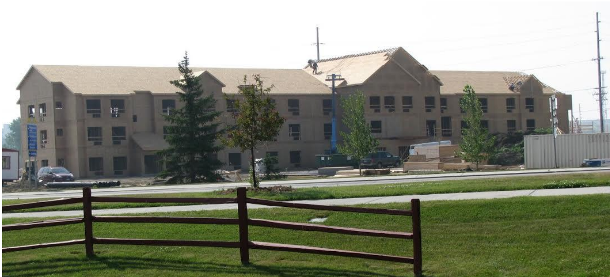
Construction of Towneplace Suites By Marriott on West 2 nd Street
