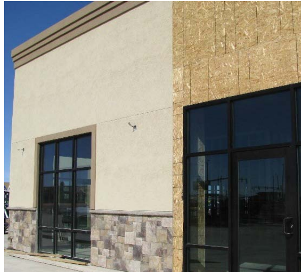
Qdoba under construction – Highway 59 and Lakeway Road
