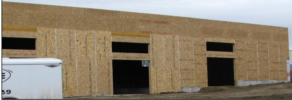
New office building being constructed on West Boxelder Road
