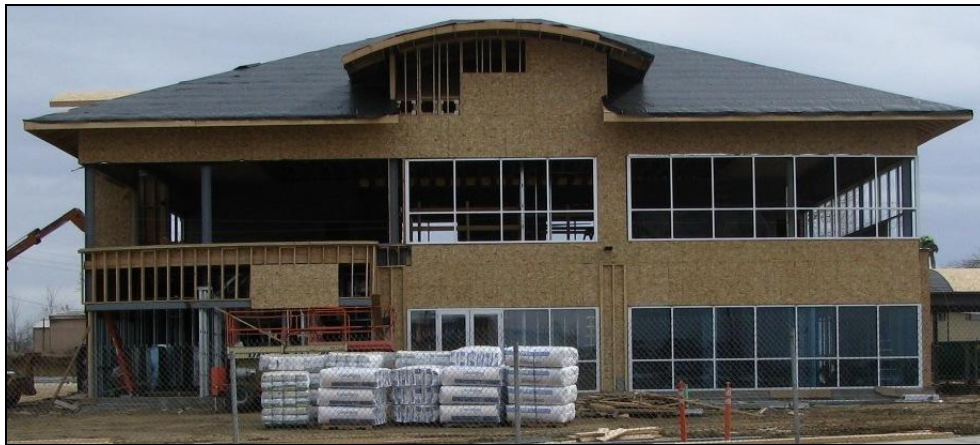
New Campco Federal Credit Union under construction on East Boxelder Road
