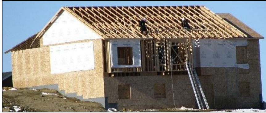
New home being built at Copper Ridge
