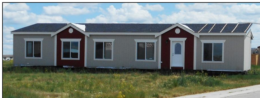
Manufactured home being placed within Morningside Estates
