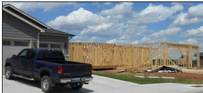
New home in framing stage at Tenth Hole Estates
